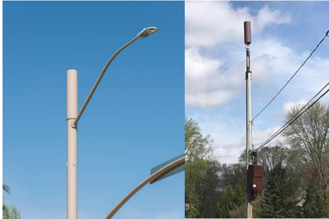
Small Wireless Telecommunication Facility photo simulation showing example of stealth antenna facility on an existing utility pole, light pole fixture, or wireless support structure. Image Credit: Crown Castle
