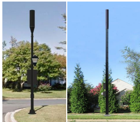
Small Wireless Telecommunication Facility photo simulation showing example of stealth antenna facility on new utility pole or wireless support structure. Image Credit: Montgomery County, Crown Castle; Crown Castle; City of Gaithersburg, Crown Castle
