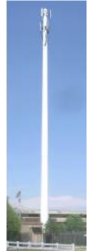
Tagging Monopole with Co-Location Using Slick Antenna
