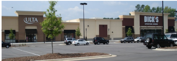
Roofline Variation and Parapet Finish
