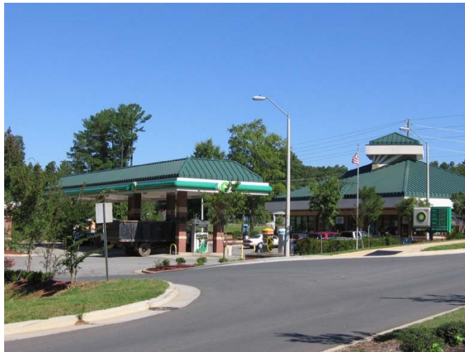
Example of Gasoline Dispenser and Canopy
