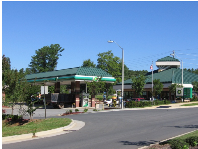
Example of Gasoline Dispenser and Canopy
