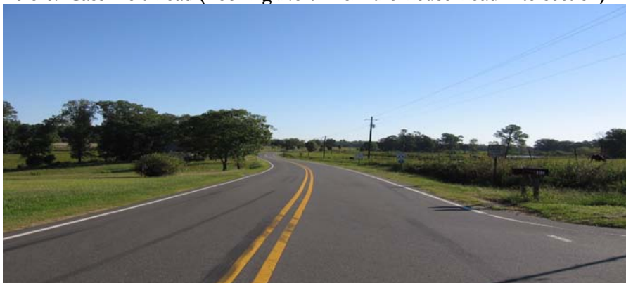
Before: Cass Holt Road (Looking North from the Rouse Road Intersection)
