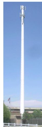
Tapering Monopole with Co-Location Using Slick Antenna
