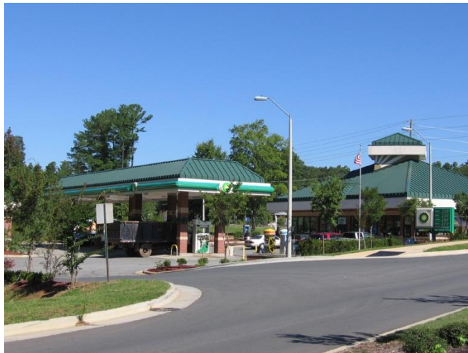
Example of Gasoline Dispenser and Canopy
