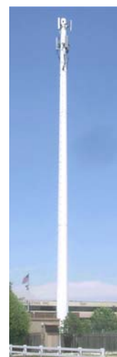
Tapering Monopole with Co-Location Using Slick Antenna
