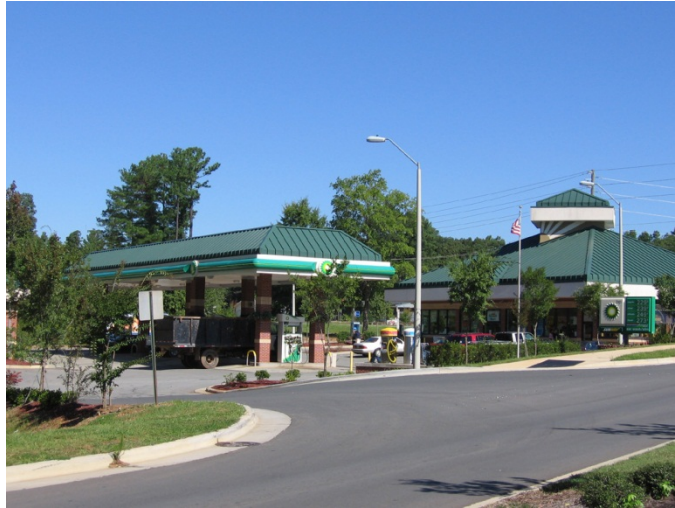
Example of Gasoline Dispenser and Canopy
