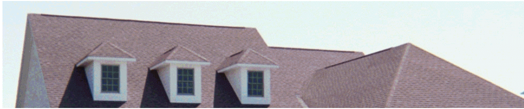
Example of: Change in Direction of Roof Ridge; Dormers and Hip Roof. [Amended Ordinance #06-04]*
