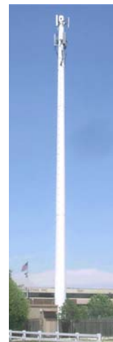
Tapering Monopole with Co-Location Using Slick Antenna
